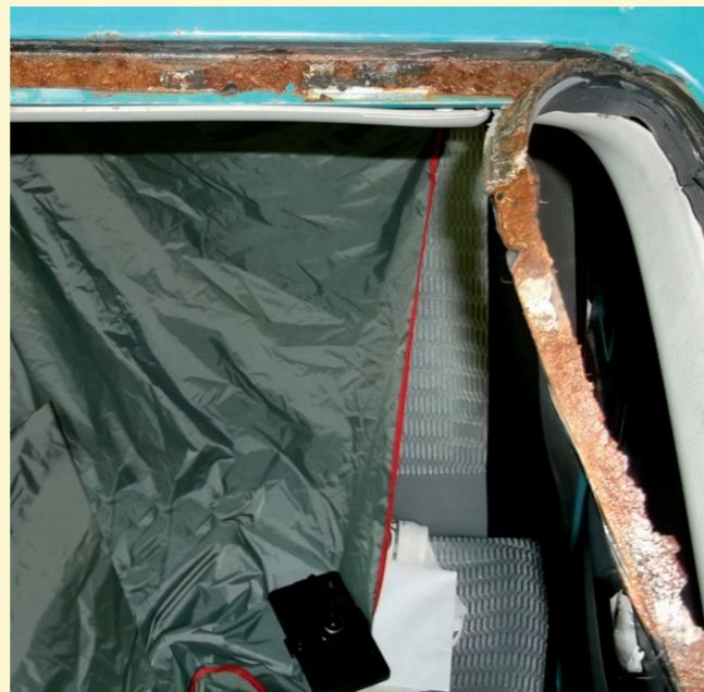
Corrosion due to lack of primer and incorrect aperture preparation
